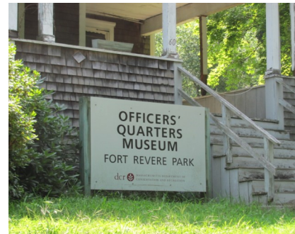
Officers' Quarters Building Farina Road 2012
